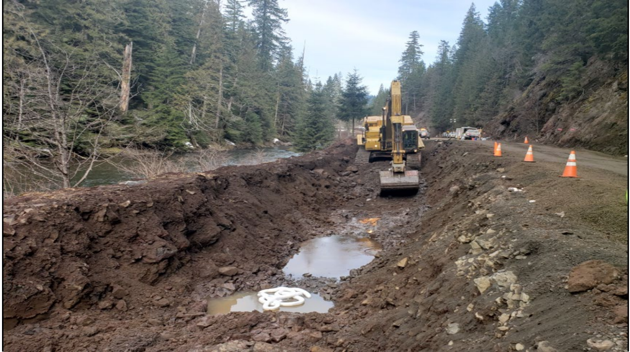
Figure 5 - Excavation to Groundwater Table - Bank Left Intact
