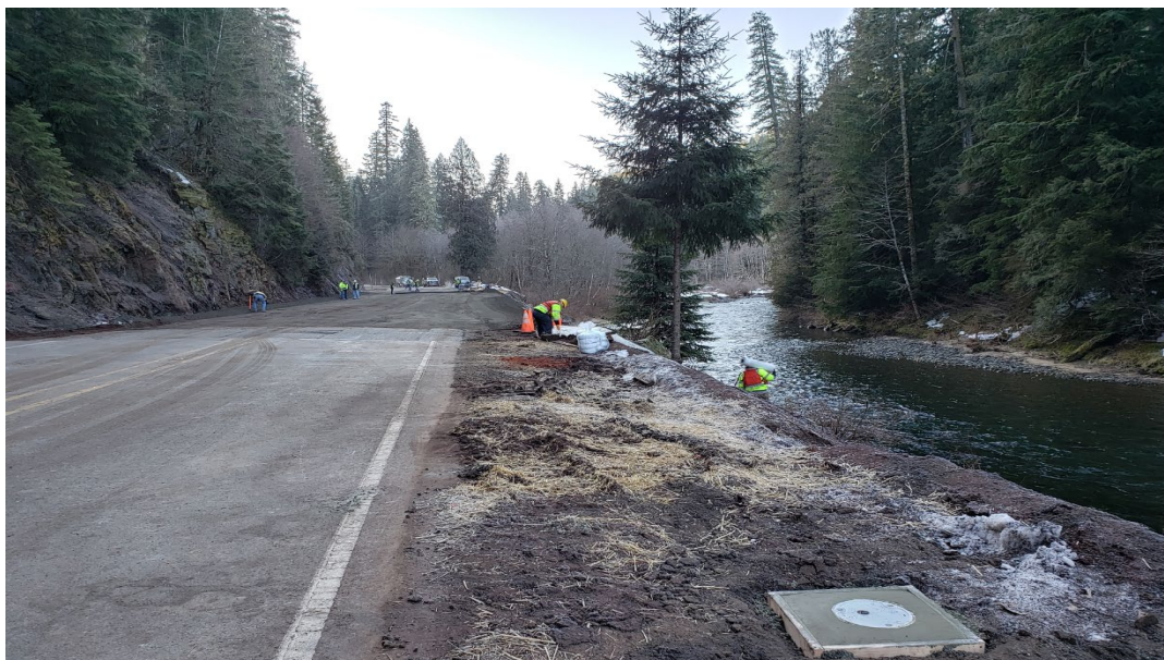
Figure 6 - Start of Highway Replacement
