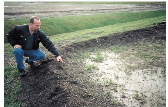
Compost berm to stabilize site.
