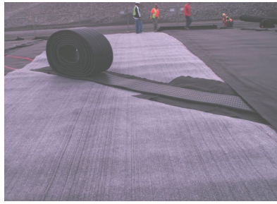
Landfill cap improvements.
